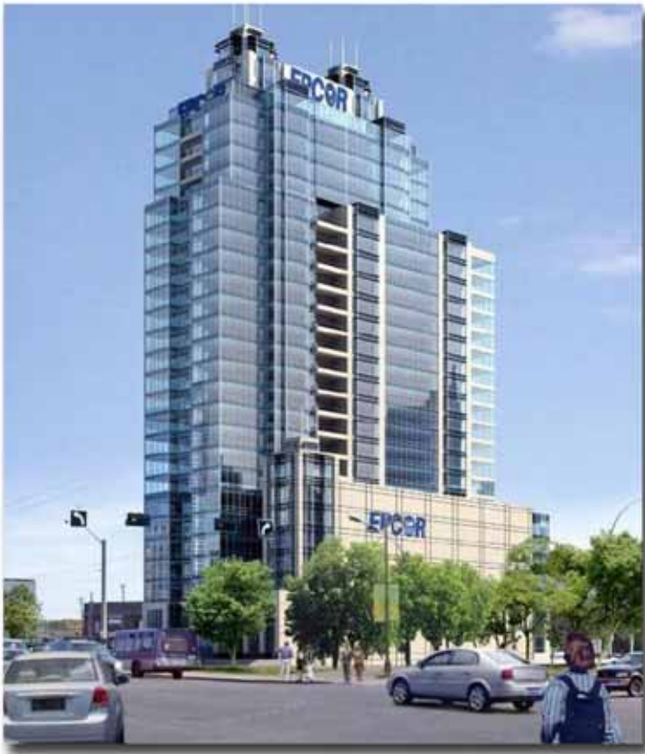
New EPCOR Tower on STATION LANDS
