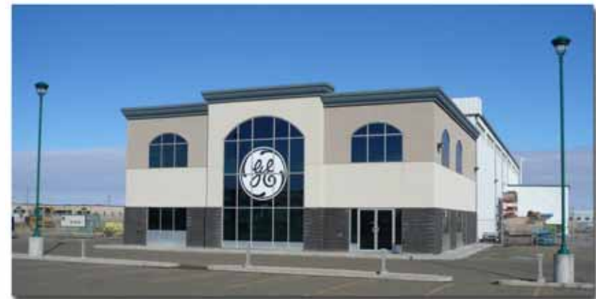
GE Turbine Building
